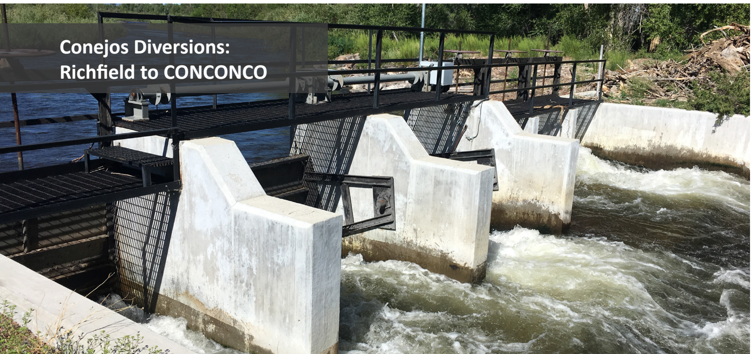
Recently completed Richfield Canal diversion dam and automated headgate on the Conejos River (photo by Peyton Valentine)
