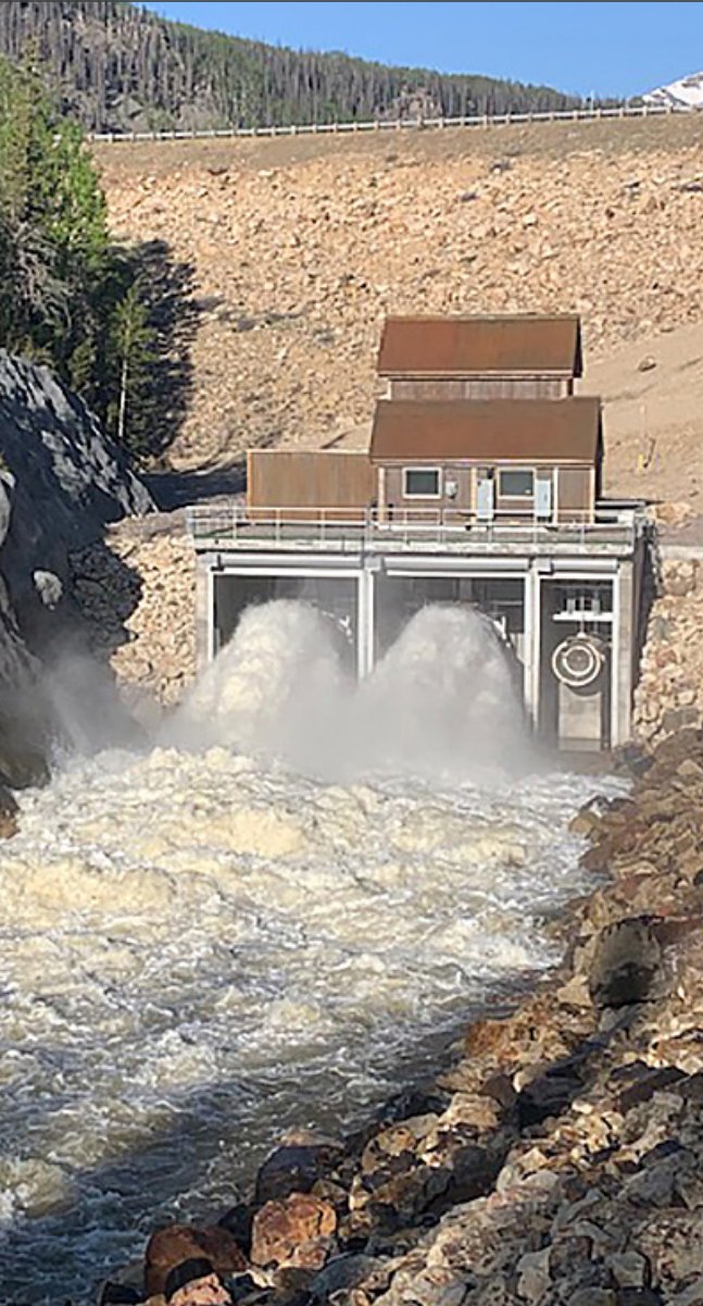
Reservoir release from the recently installed Rio Grande Reservoir outlet works (photo by Rob Phillips)
